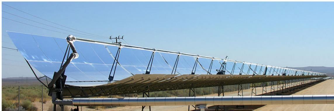
**Figure 2.11** Parabolic trough collectors are used to generate electricity in southern California. (credit: “kjkolb”/Wikimedia Commons)
